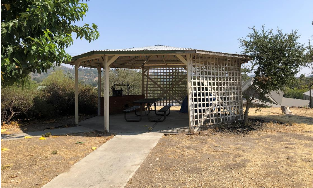
Existing gazebo to be removed
