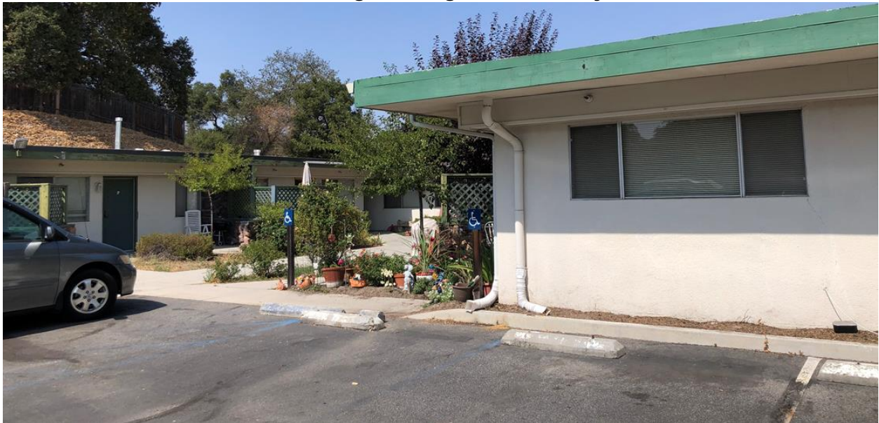
View looking at Manager's Unit/ Courtyard
