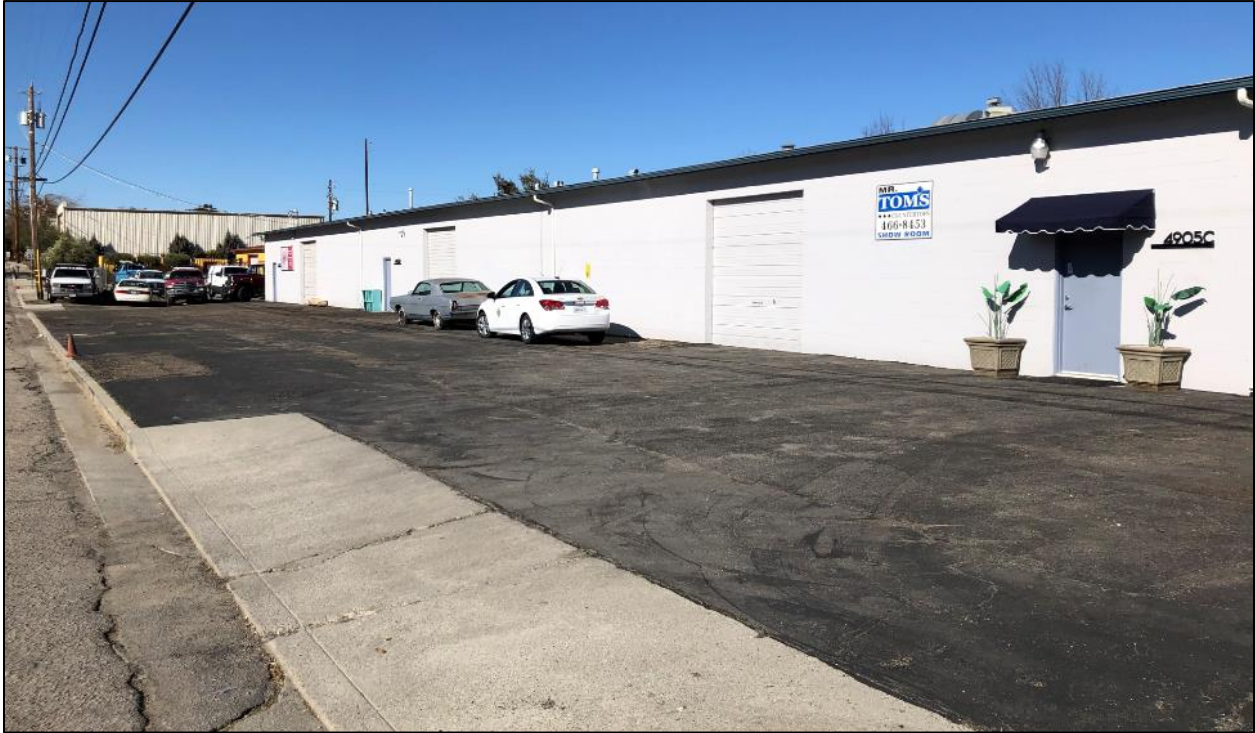
View of existing parking lot
