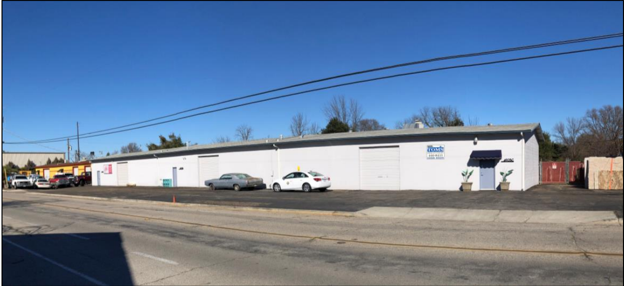
Overall site view
