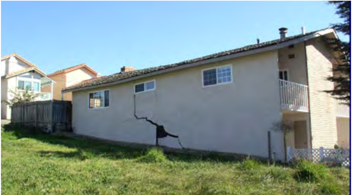
Damage to a home in Oceano caused by liquefaction resulting from the 2003 San Simeon Earthquake.
