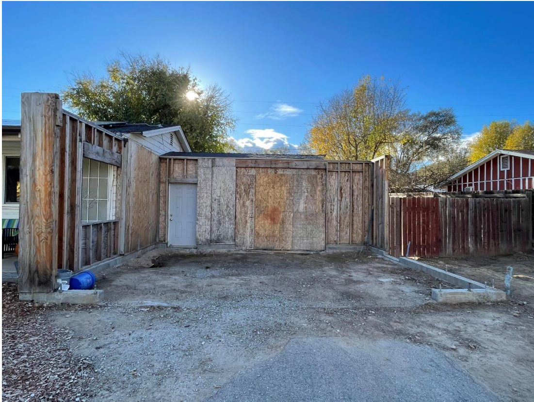
Existing partially-completed garage
