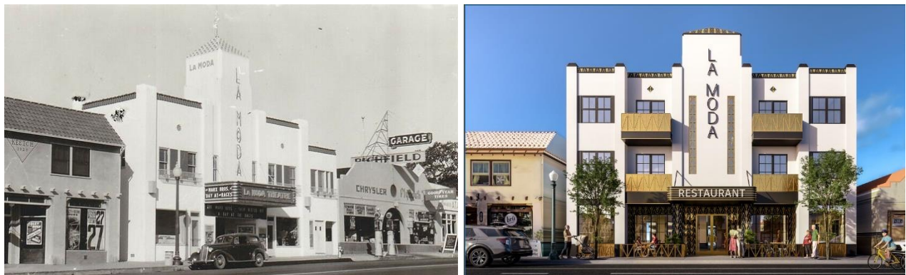
Image of the Atascadero Playhouse (on the left) compared to the rendering proposed mixed use structure from El Camino Real.
