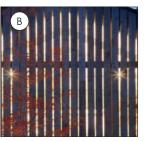
RAINSCREEN SYSTEM VERTICAL METAL PLANKS BOARDS SIMULATED WEATHERED WOOD TEXTURED FINSH
