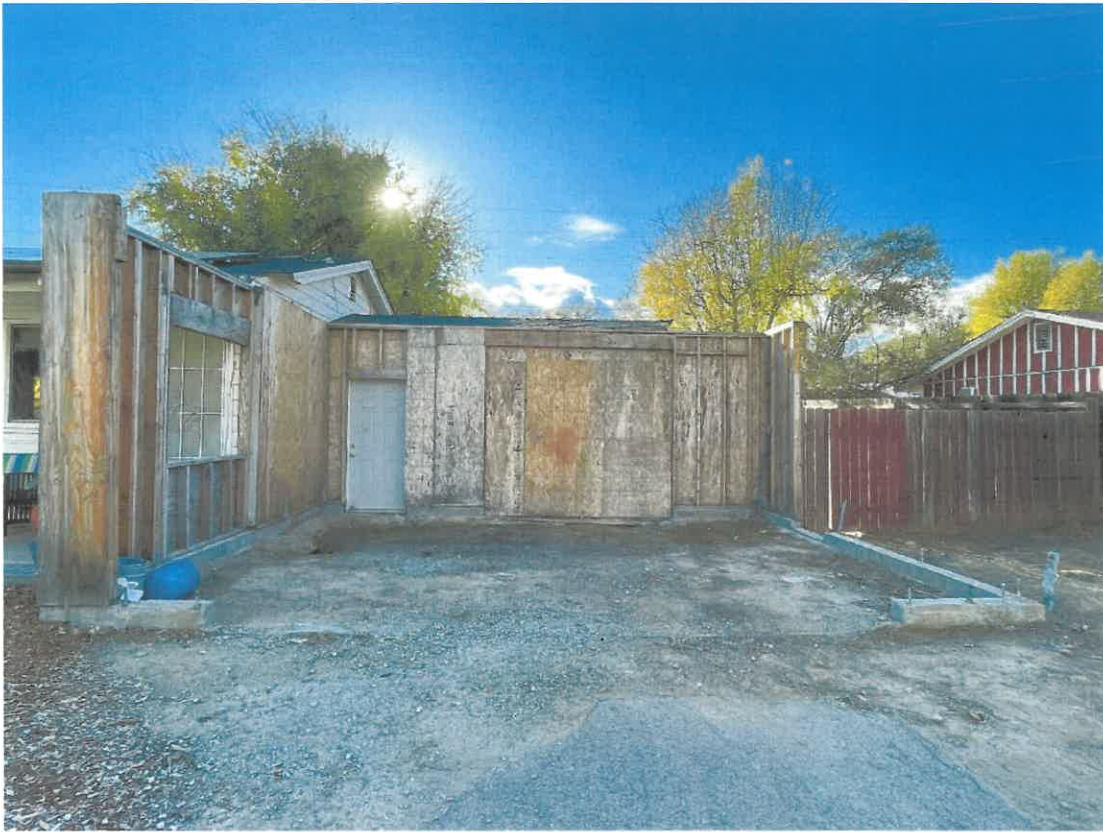
Existing partially-completed garage
