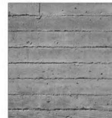
CONCRETE: BOARDFORM
