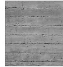
CONCRETE: BOARDFORM
