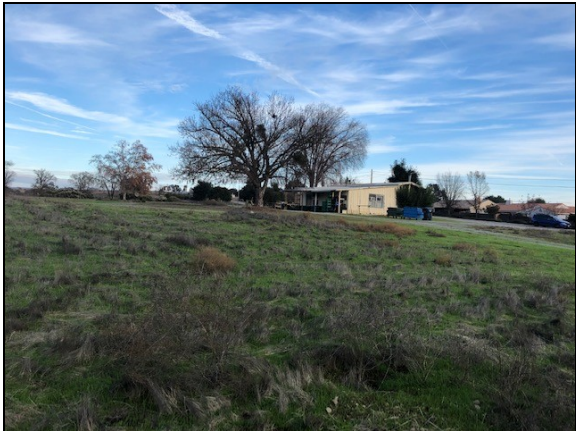
Picture 9: Looking southeast at the building on the Subject Property.
