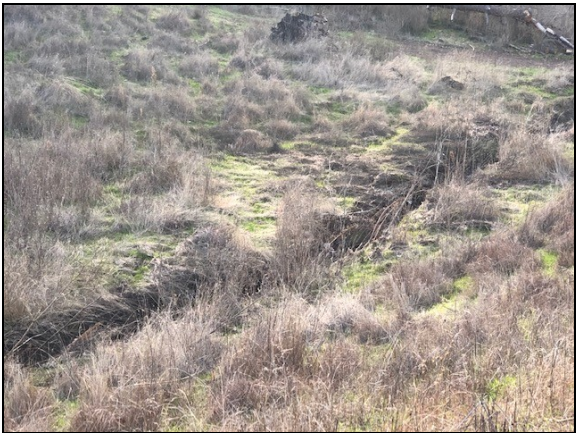
Picture 30: Stormwater drainage on the northern parcel.
