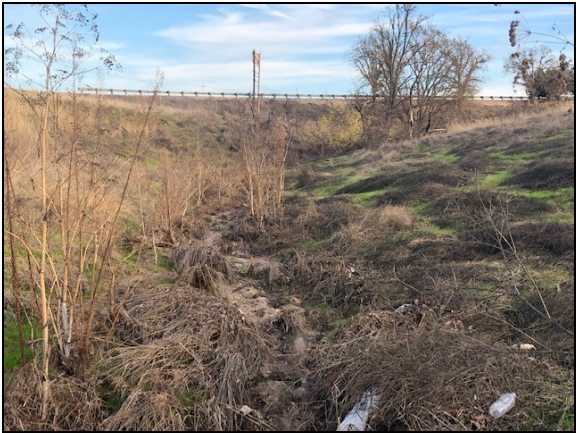
Picture 28: Stormwater drainage on the northern parcel.
