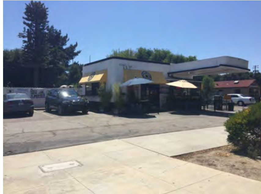
Proposed coffee shop to be demolished.
