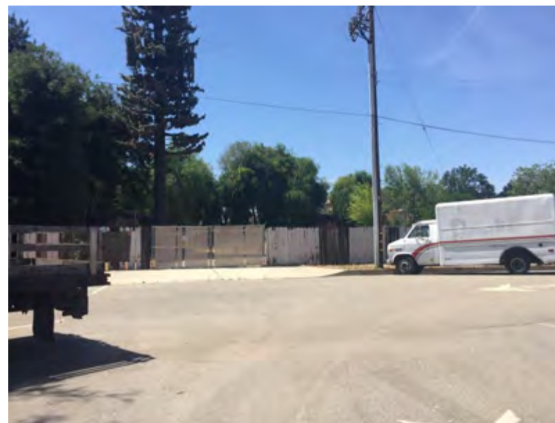
Unmanned Wireless telecommunication facility.
