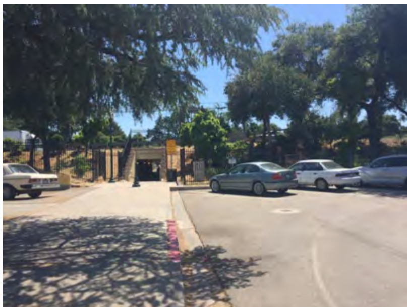
View of pedestrian tunnel along Atascadero Avenue (Atascadero Mall)
