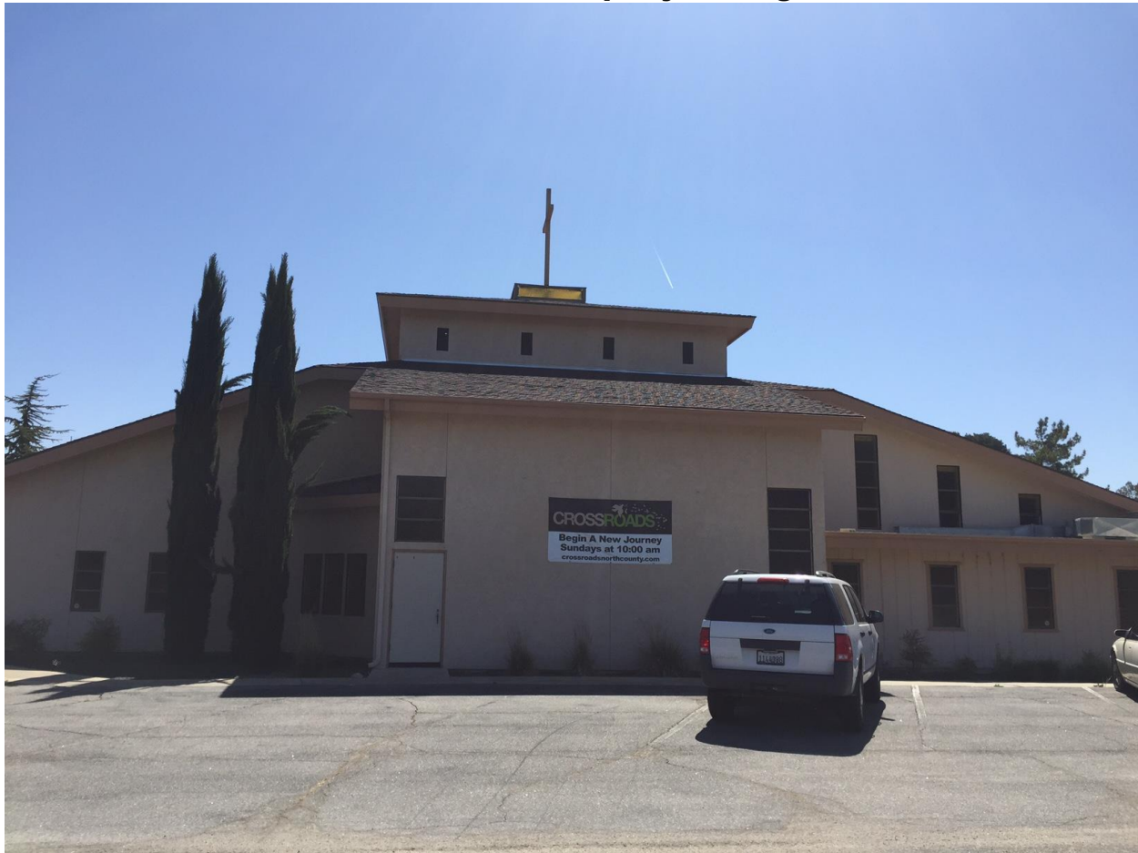
View from Front of Property looking East
