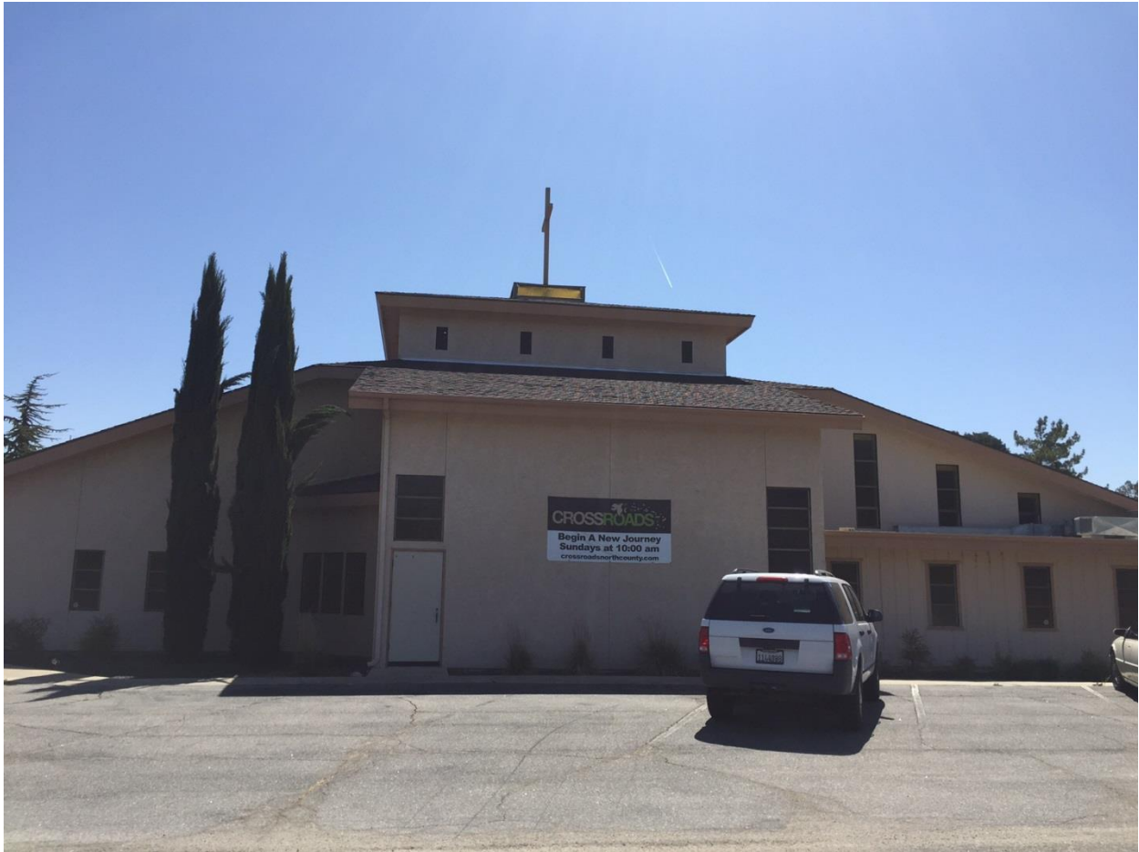
View from Front of Property looking East
