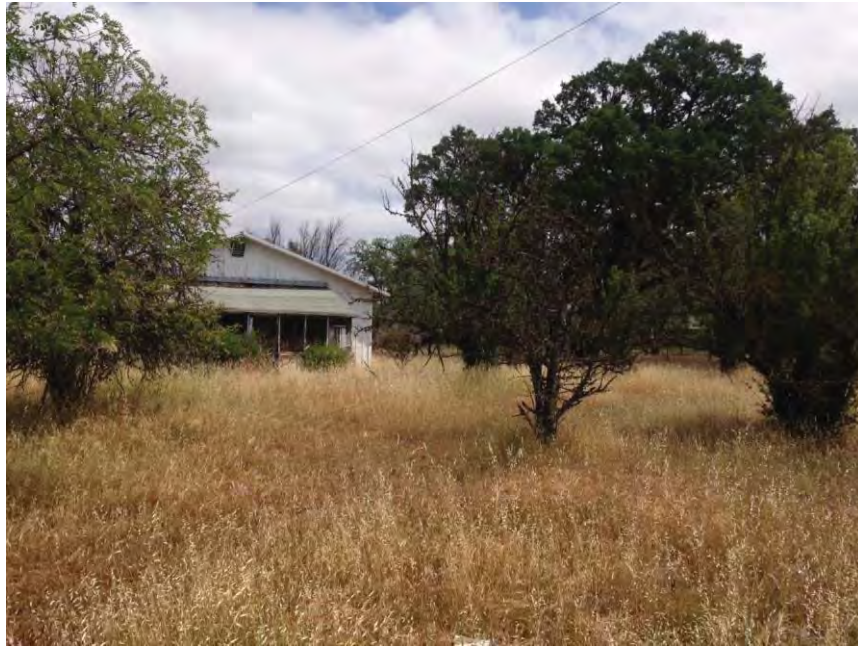
View of existing vacant building from El Camino Real.
