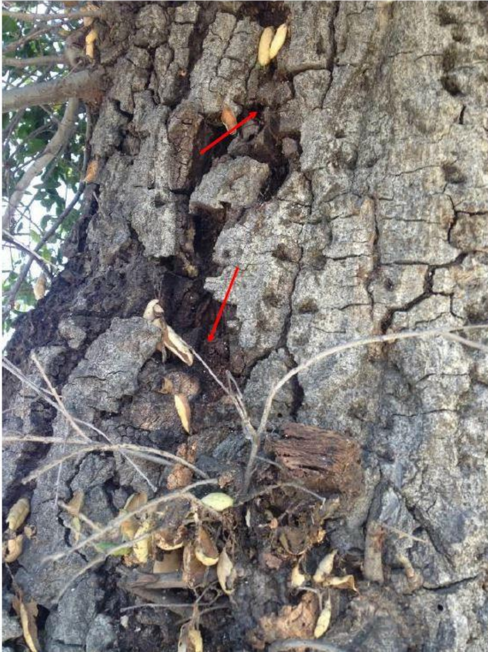
Photo 2: Showing external decay and cracking in main trunk at base of dead leader
