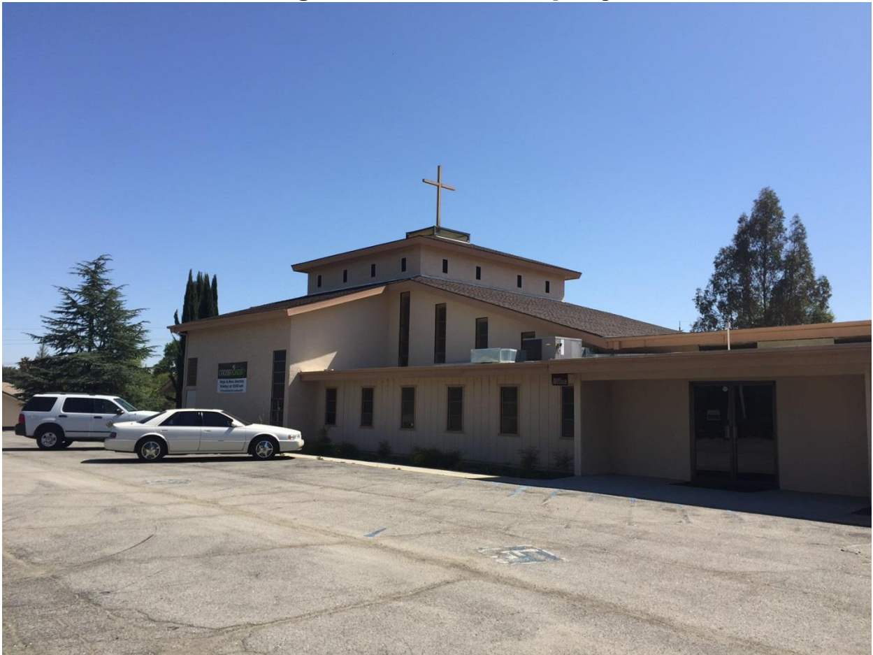
View looking Northeast from Property at Front
