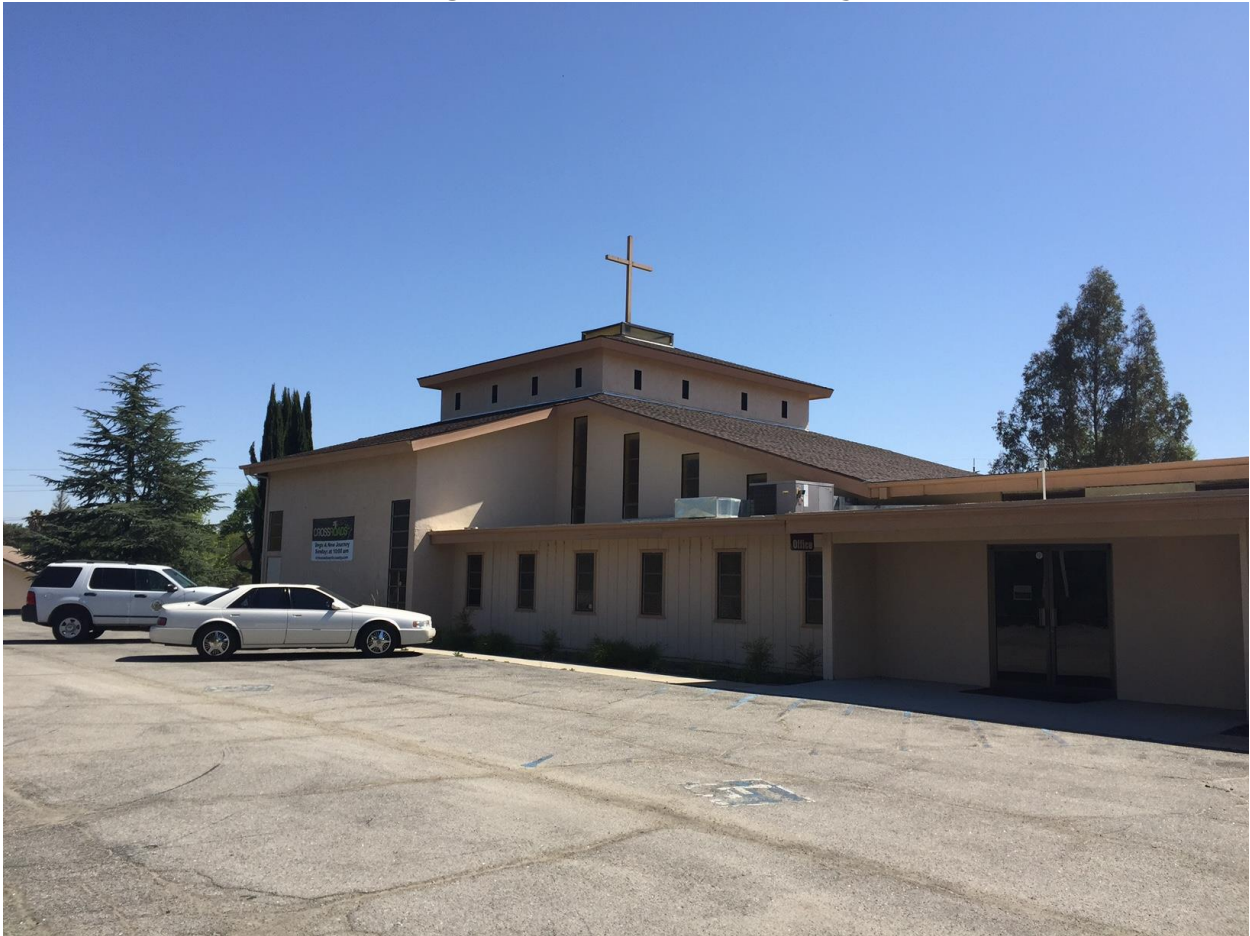
View looking Northeast from Property at Front
