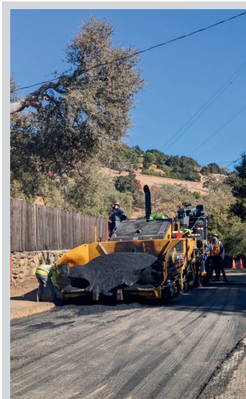
Monita Rd. Rehabilitation
