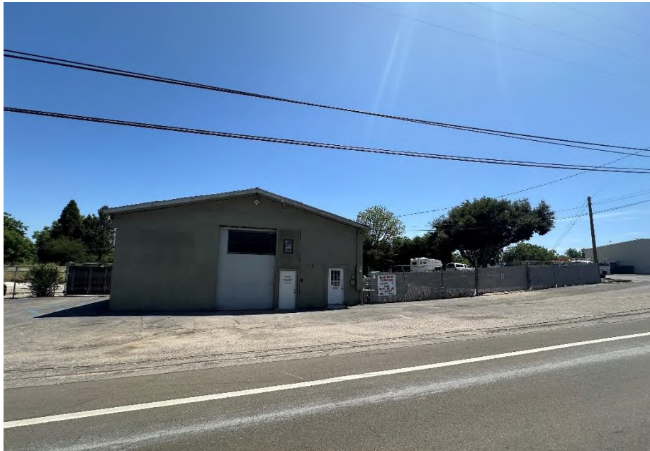
View from Traffic Way – Industrial Building and Fenced Parking Area
