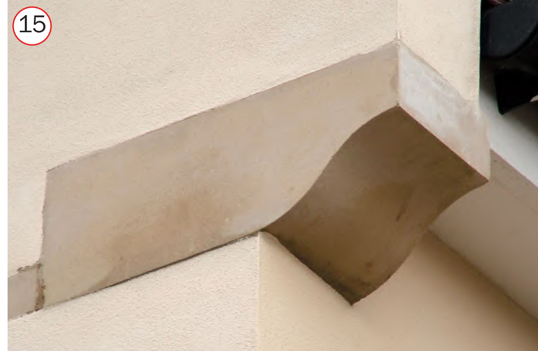
ROOF DETAIL: CAST STONE CORBELS
