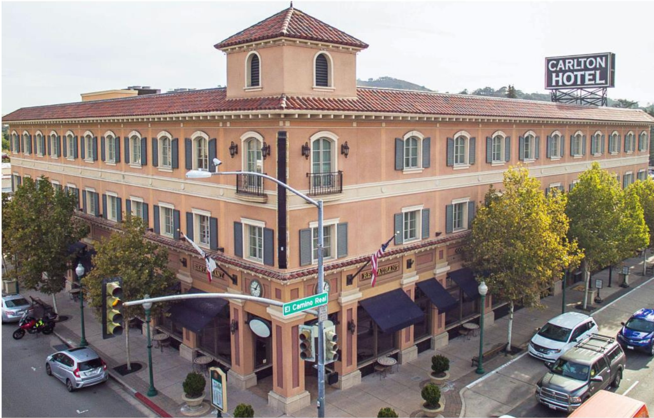
Elevated Corner View, North and West Facades, from the intersection of El Camino Real and Traffic Way.
