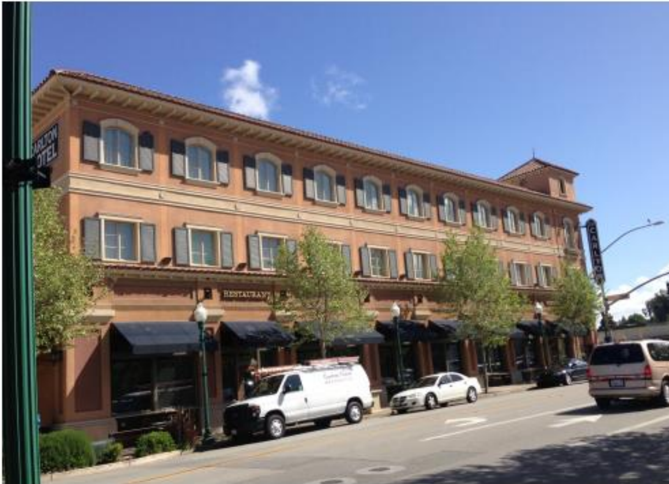
Front View, North Façade, from Traffic Way
