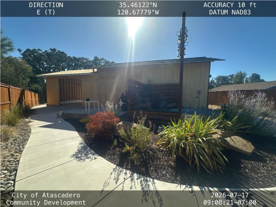
West Façade of (E) Garage with As-Built Addition
