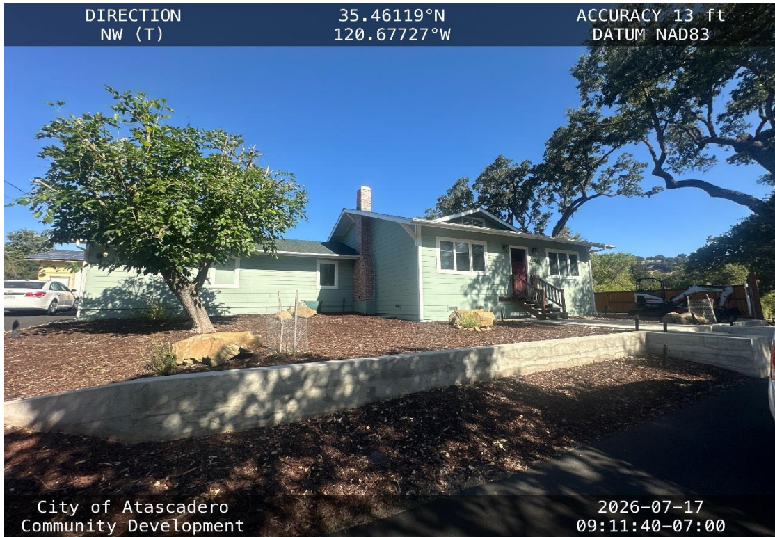
(E) Colony House / Primary Structure
