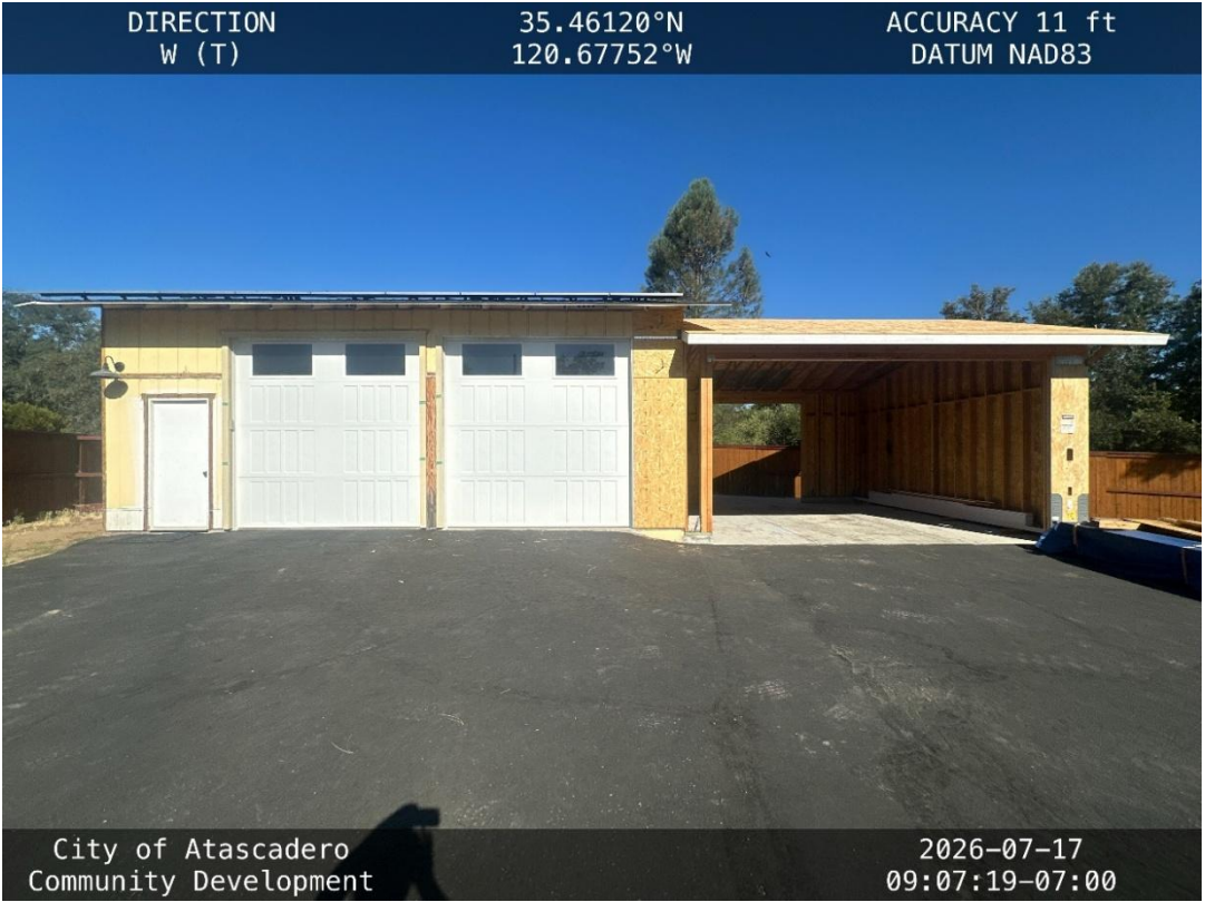
East Façade of (E) Garage with As-Built Addition
