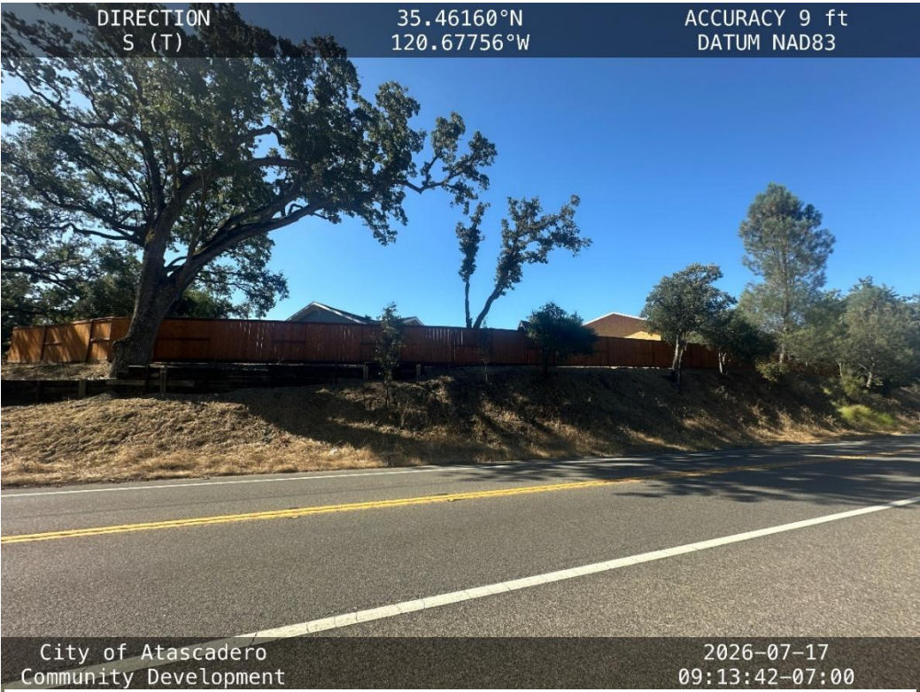
View of (E) Garage with As-Built Addition from Morro Road
