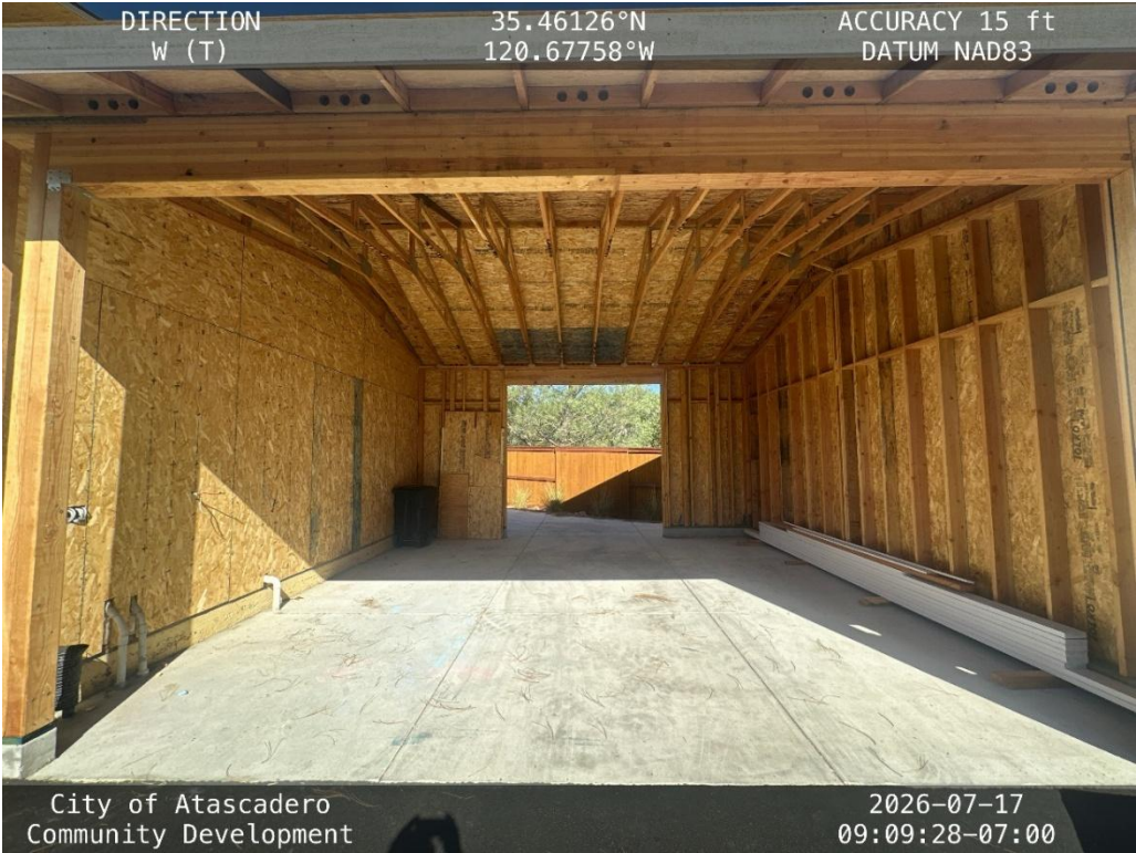
Interior of (E) Garage with As-Built Addition
